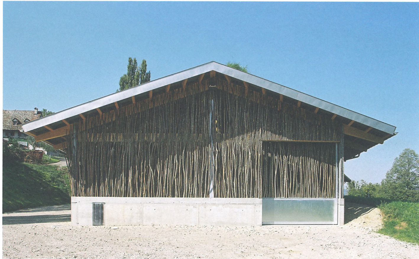
The dairy barn at Schönenberg Farm blends into its hillside site with a sod roof and hazel branches for walls.
